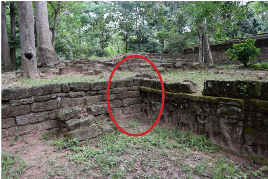
Figure 17: Juncture between sandstone and laterite building phases blocking bas-relief, ATTS008 (Terrace des Hamsas), Royal Palace
