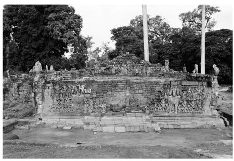
Photo 1: East facade of the North Stairway of the Terrace of the Elephants in 1997 during the restoration works. Note that M3 has been temporarily dismantled for complete anastylosis, revealing entirely the east side of M2. (©EFEO)
