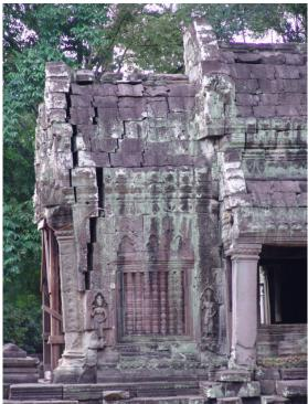
Fig. 1: Typical examples of the structural failures of the corner or end parts of monuments.
