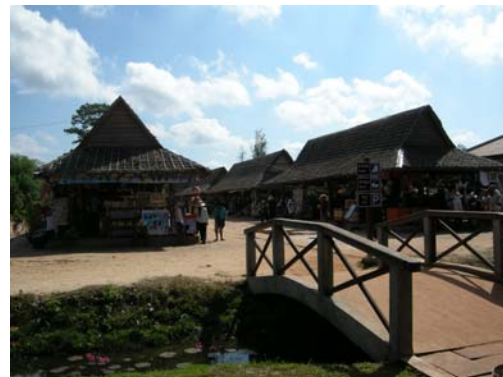
Shops after development
