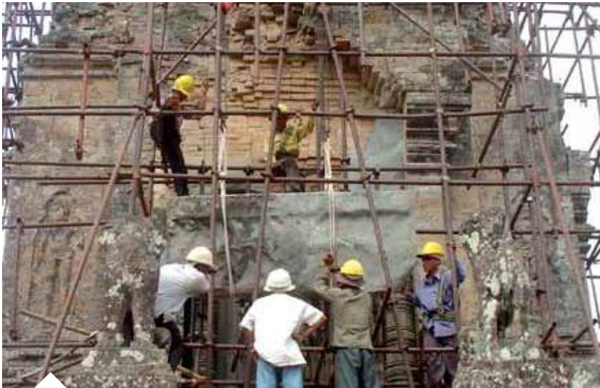
Repositioning of a fallen lintel to its original place
