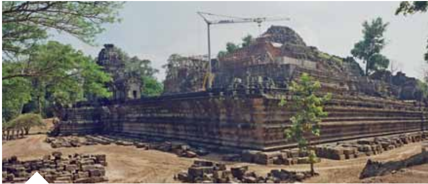
Overview of the work site
