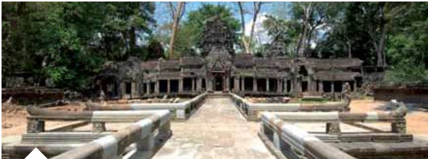
Causeway between the third and fourth enclosures, facing west (after work)
