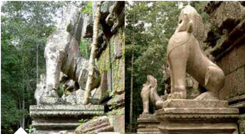
Shape of the lions before and after the restoration works
