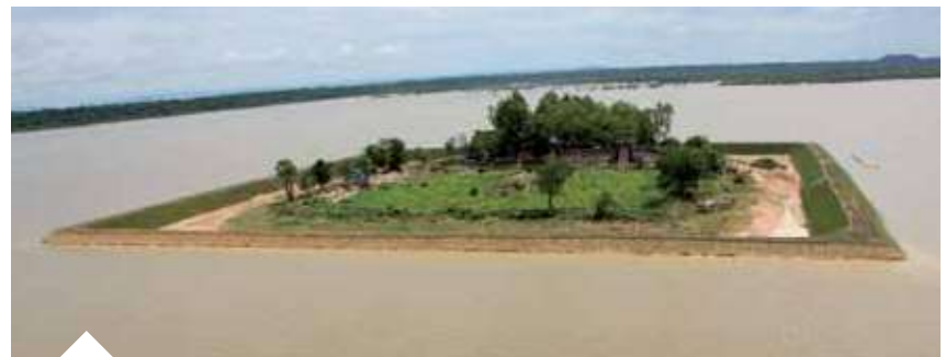
Temple protected by temporary dike during restoration
