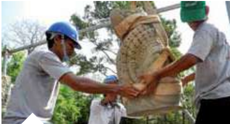
Students replacing cement heads with newly carved sandstone replicas, South Gate of Angkor Thom
