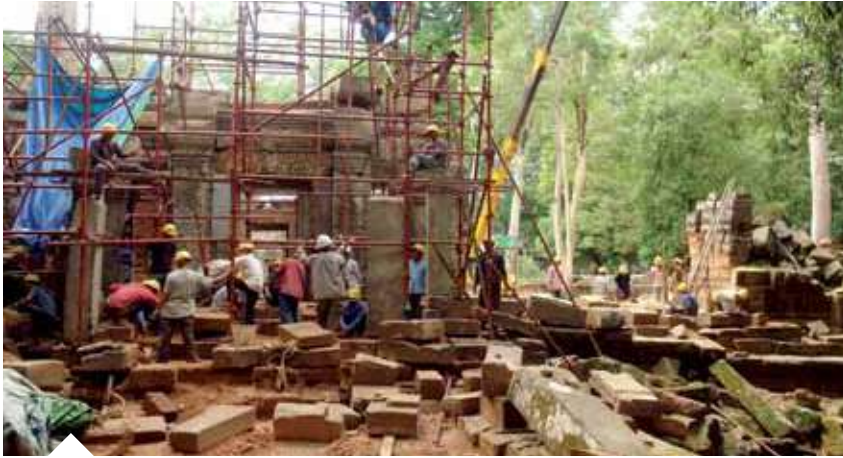
Western Gopura of the fourth enclosure, facing west (during work)
