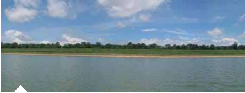
View of 560 meters of the West Baray dike after restoration
