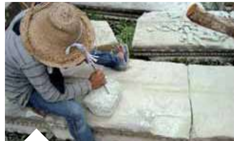
Chiselling of the surface of added new pieces of sandstone blocks to the upper staircase
