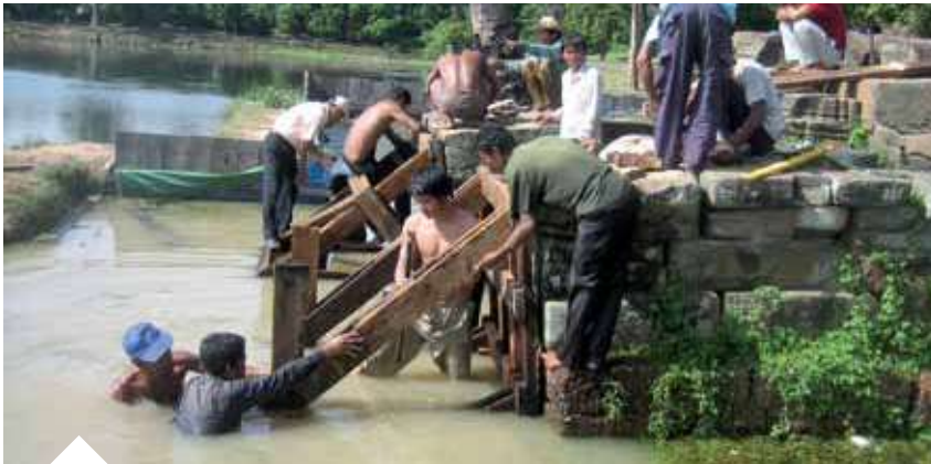
Dismantling work at the pier
