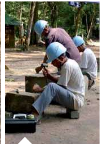
Workers carving sandstones for repairs
