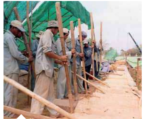
Compacting the soil on the western causeway, 2005
