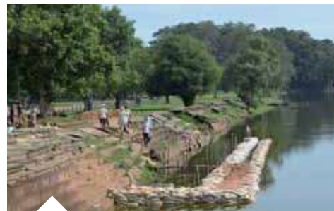
Restoration of the moat embankment, extension span, 2012 - 2014
