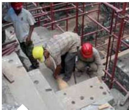
Putting stone components back to original positions at eastern exterior gopura
