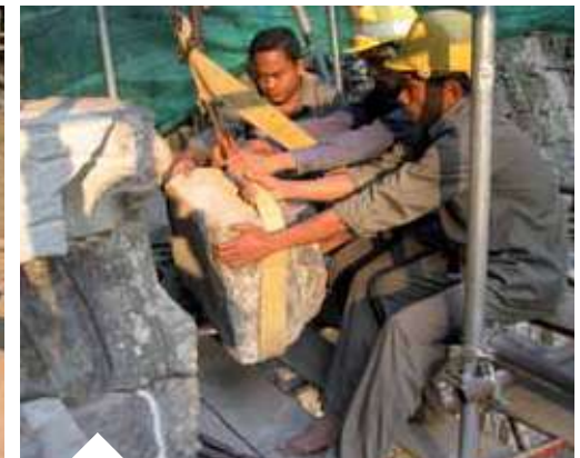
Resetting a stone to its original position
