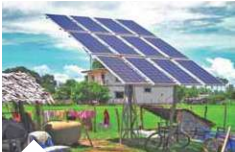
Solar panel station
