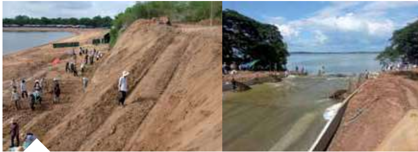
Restoration work on the western dike
