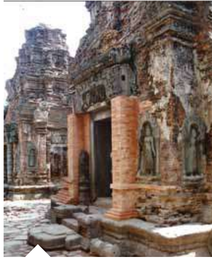
Same shrine after the intervention, 1994
