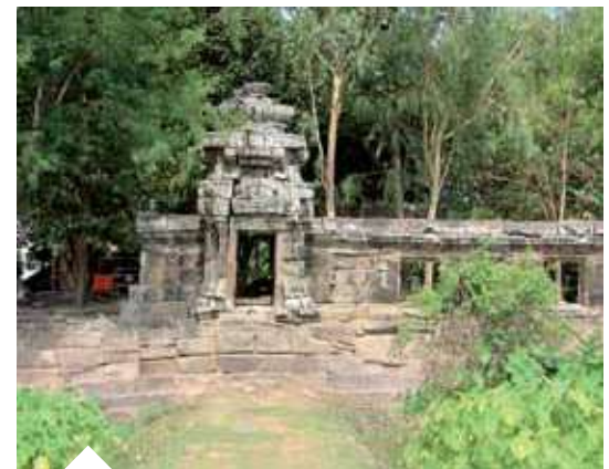
Axial pavilion, eastern enclosure dismantling
