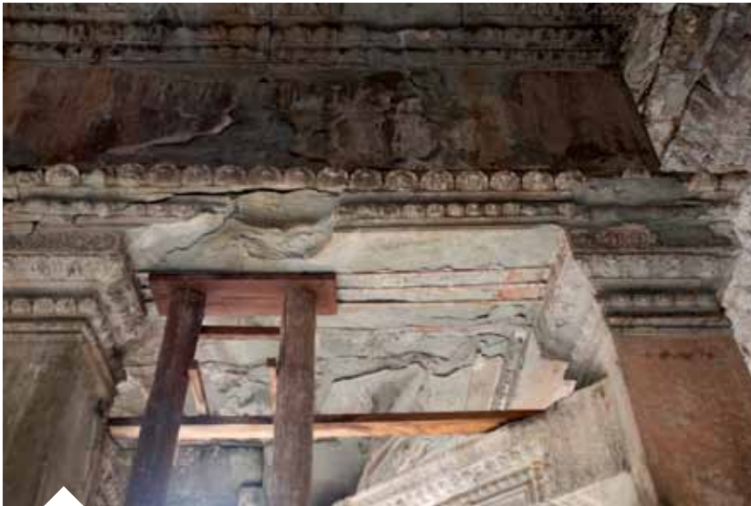
Provisional roof structure support - Angkor Vat
