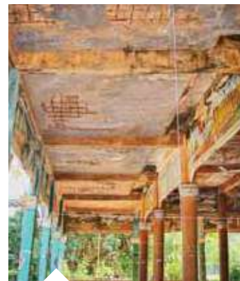
Dilapidated state of the Vihear and wall paintings
