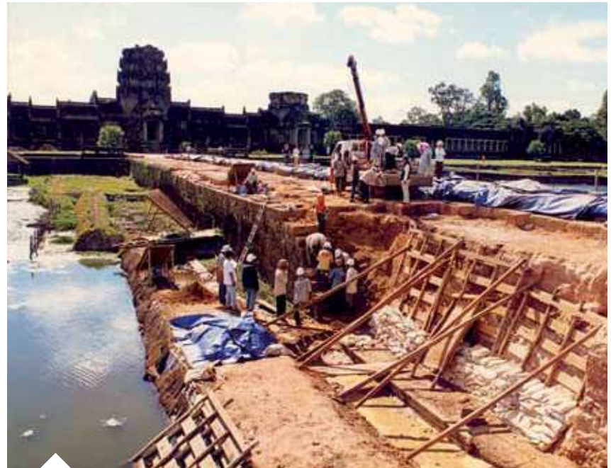
Dismantling of the western causeway, 2000
