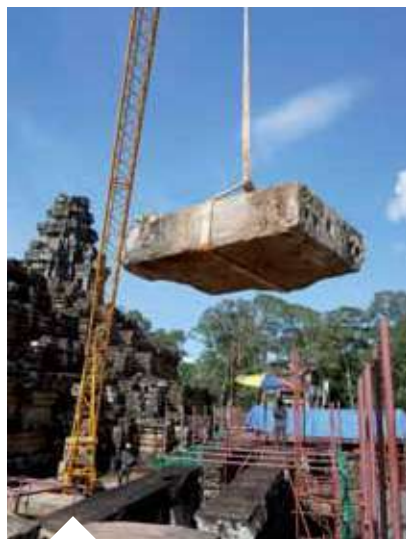
Dismantling process of corner tower of southwest corner, second tier platform
