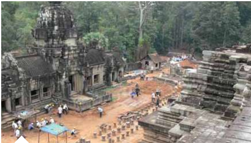
Restoration of the eastern courtyard, first tier
