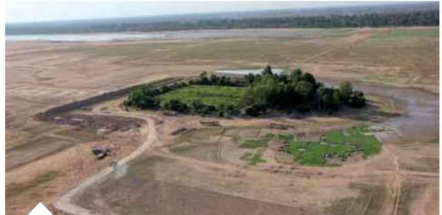
Construction of the dike for the work site protection
