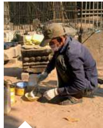
Preparing structural adhesive for stone repair
