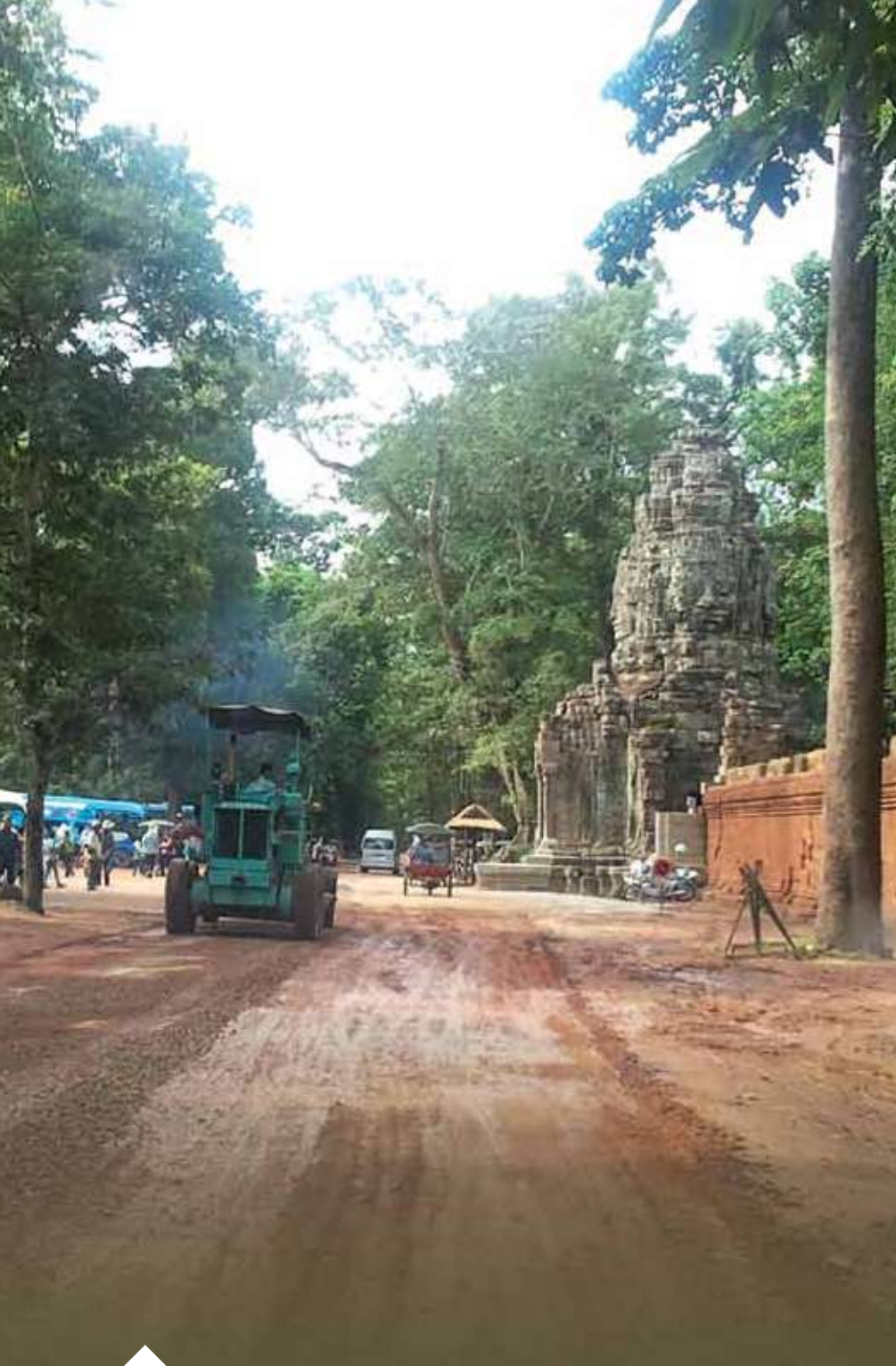
Road renovation - Ta Prohm
