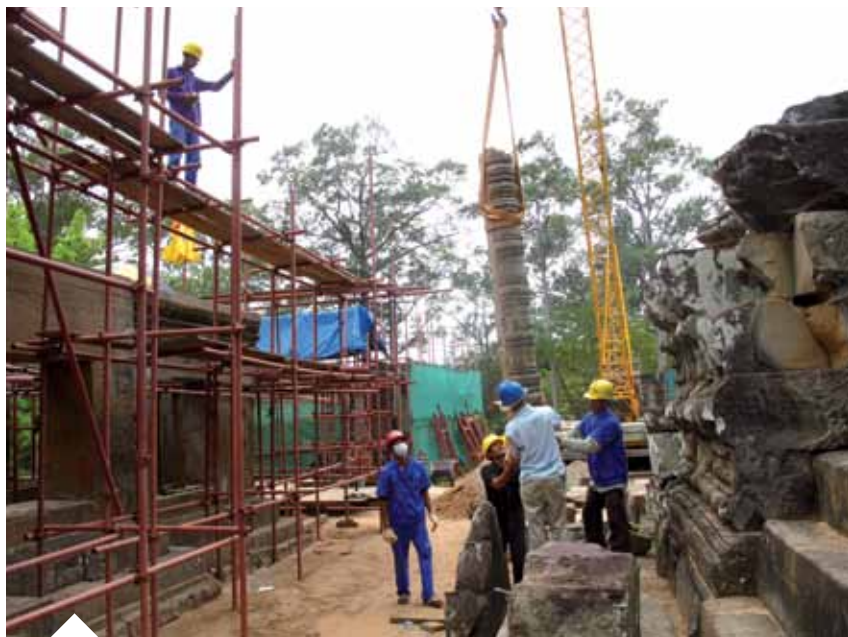
Assembling a colonnette on southern interior gopura
