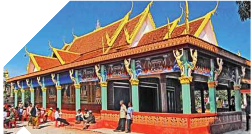
Overall view of the Vihear after restoration
