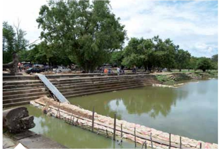
Panoramic view of the restored first span of moat embankment (2009 to 2011), and of the ongoing works (2012 and expected until 2014)
