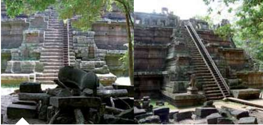
Shape of the staircase before and after the restoration works
