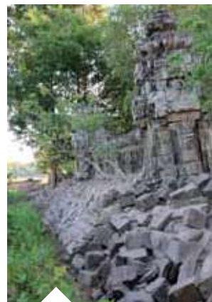
Eastern façade before dismantling
