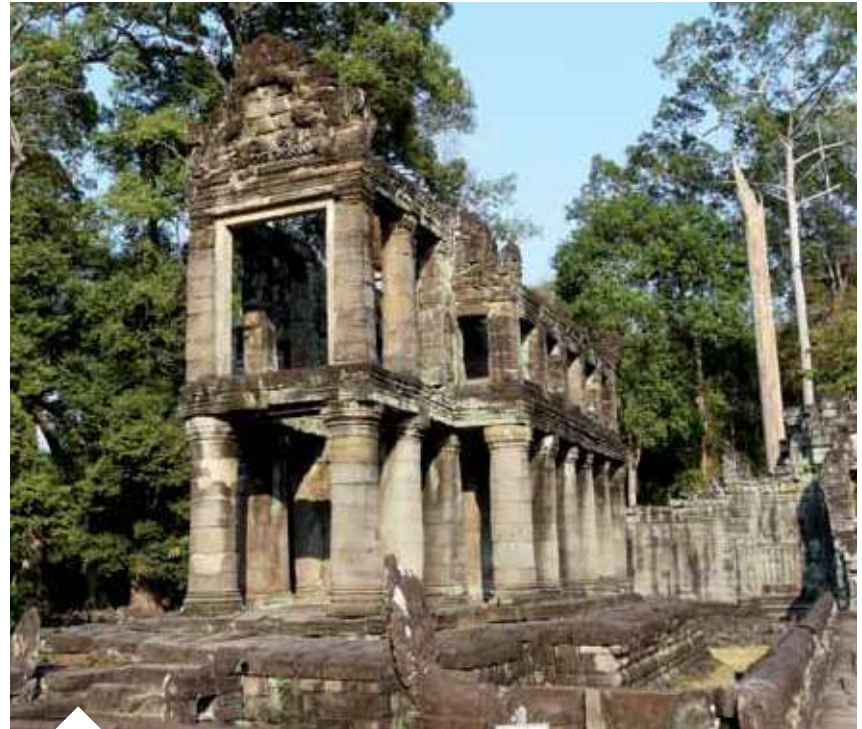
Ongoing implementation of a conservation and stabilization plan for a unique two-story pavilion
